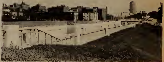
Section III line construction as seen from the Atherion Street bridge.
